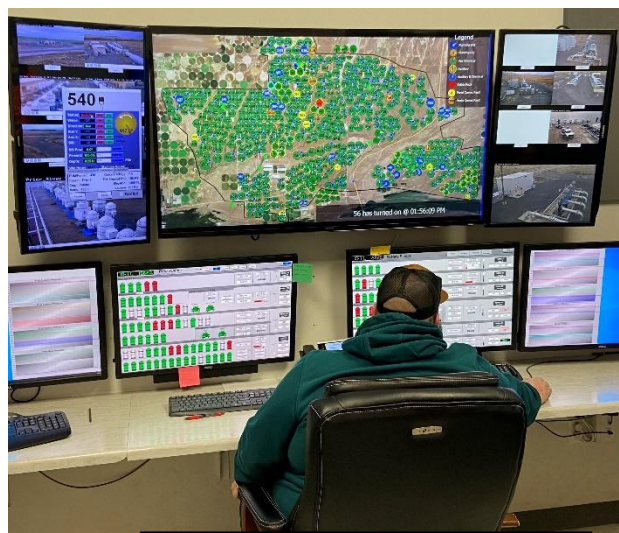
Figure 10. Irrigation control station Agri-Northwest Oregon. Over 500 centre pivots are controlled here 24/7. Author's own photo. See Case study 3 in appendices.
